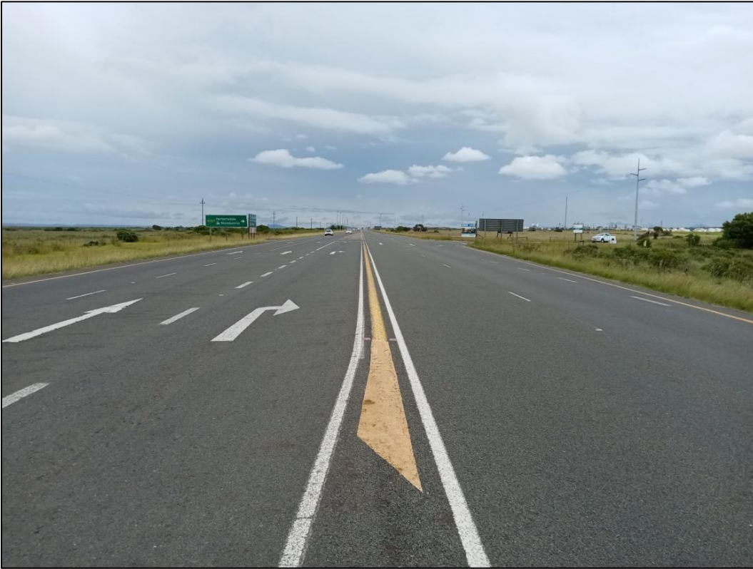
Figure 3-2: N2 / R327 Intersection (looking west along N2 towards R327)
