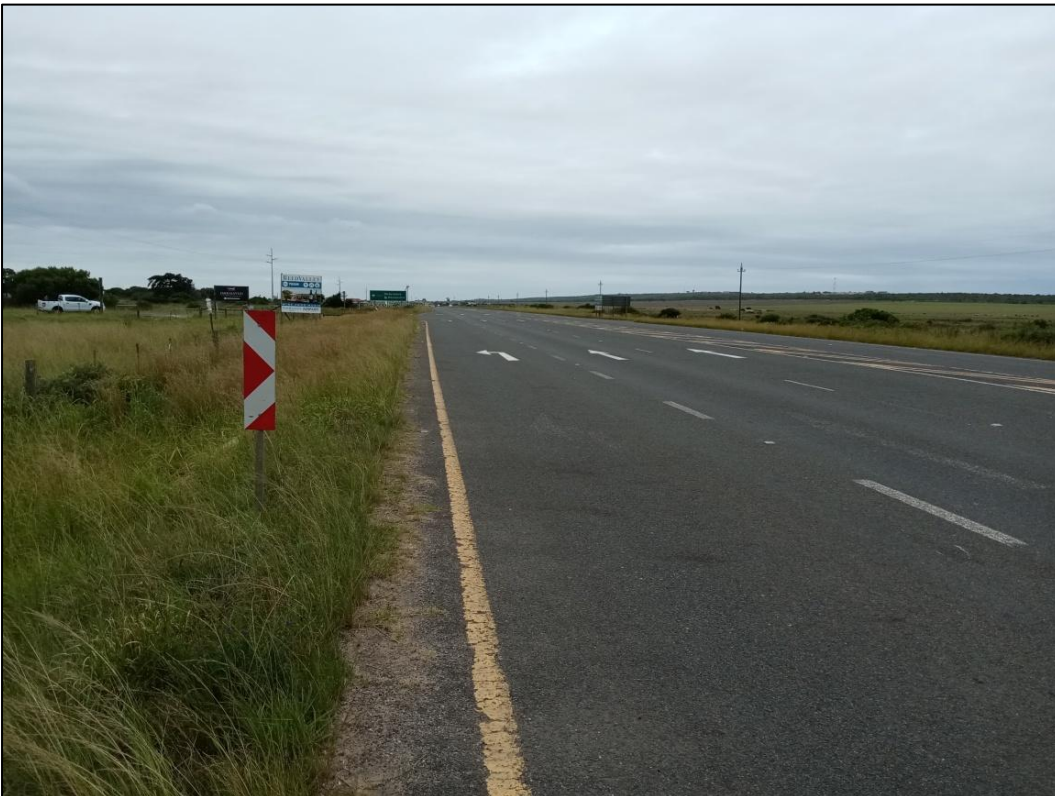
Figure 3-3: N2 / R327 Intersection (looking east along N2 towards R327)
